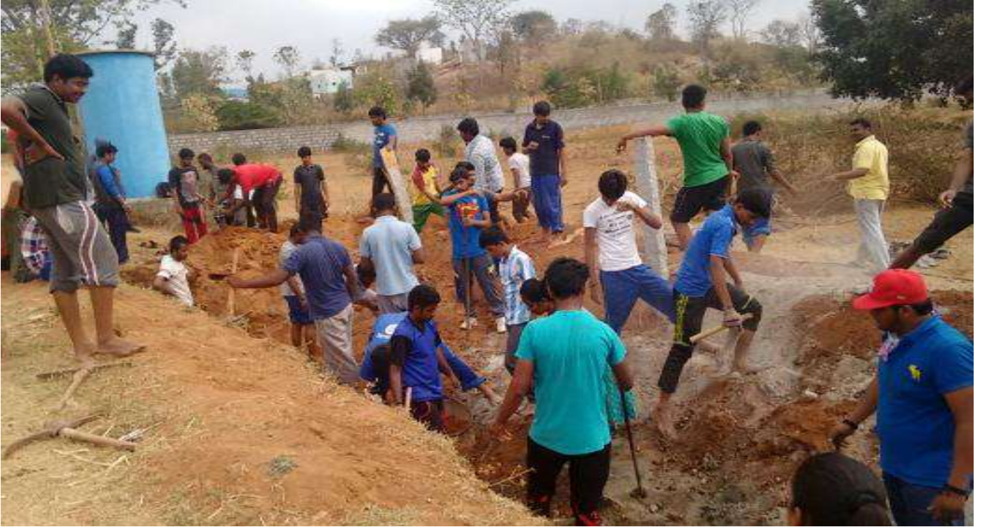
Shramadhana, Construction of check dam.
